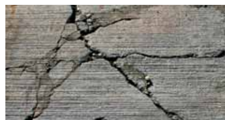
C CRACKED CONCRETE LANDING
