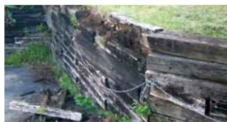
B ROTTING RAILROAD TIES
