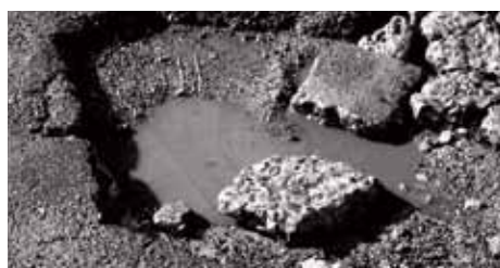
A POTHOLES IN ASPHALT DRIVEWAYS
